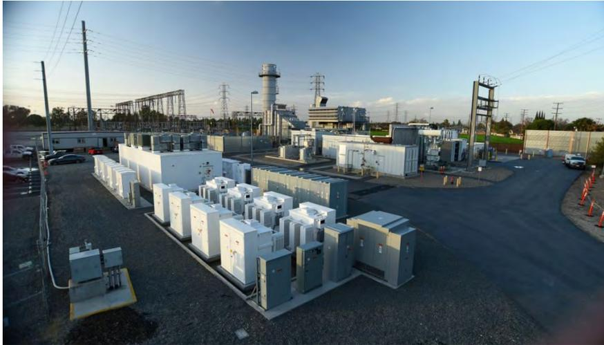
The system is designed to immediately supply power when needed; the first response is discharging the battery while starting up the gas turbine to provide the required energy. SCE estimated that the hybrid system will reduce the greenhouse gas emissions of the peaker plant by 60% over its life time.
