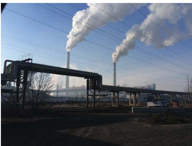
CHP#3 coal-fired thermal power plant, with district heating steam pipes in foreground, and coal loader in background.
